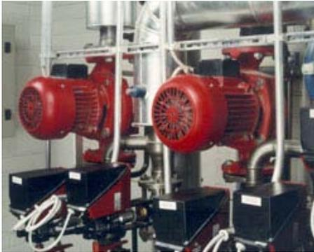
Electronic adjustable speed drives can control flow rates in pump and blower applications, eliminating throttling valves and dampers, with energy savings of 20%!
